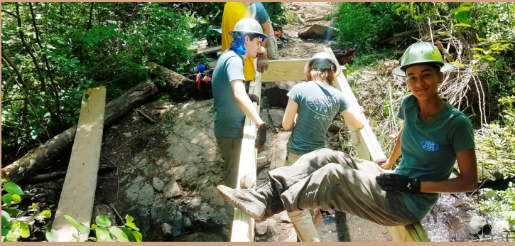
Connecticut trail crew completing new footbridge on NET.
